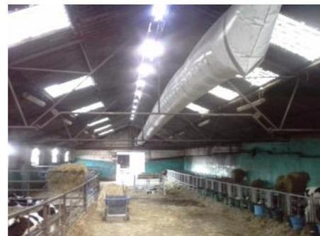
are purchased based on the shed’s dimensions. These ensure that the total volume of air in the shed is changed 4-6 times every hour and that air is spread evenly over the stock at a speed that will not chill them.
